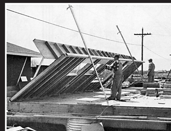
▲ Two Proctor Wall Jacks lift a sheathed wall with finished soffit in Chicago, Illinois.
